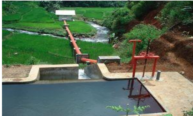
Figure 3: Pen stroke for Pico-hydro system
